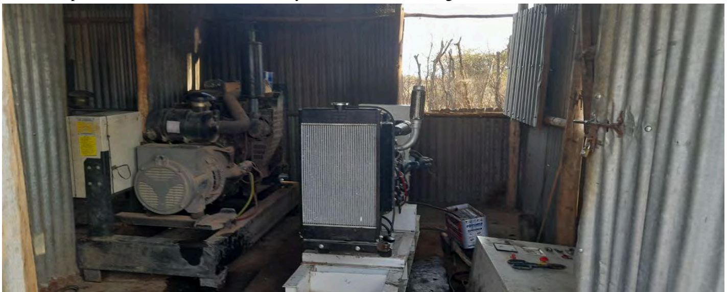
Fig. During Generator installation
