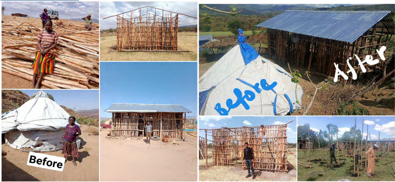
Figure: Shelter Construction in Konso
