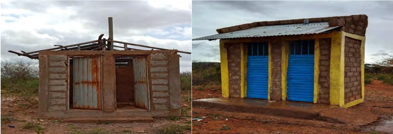
Fig. before and after rehabilitation of latrine
