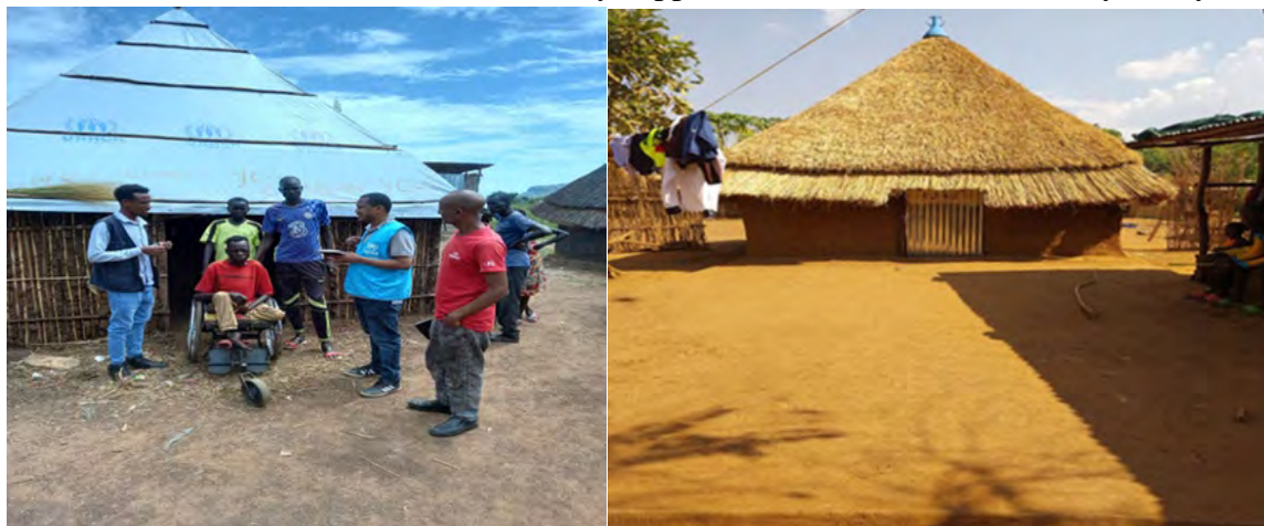
Fig. T-Shelter constructions at Gambella Operation
