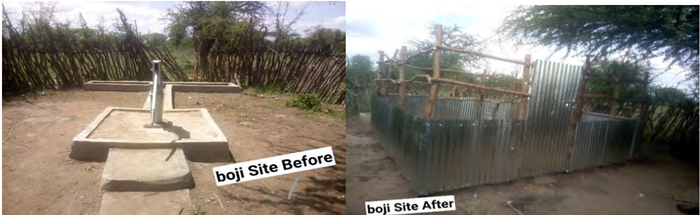
Fig. Rehabilitation of Shallow well Before and after
