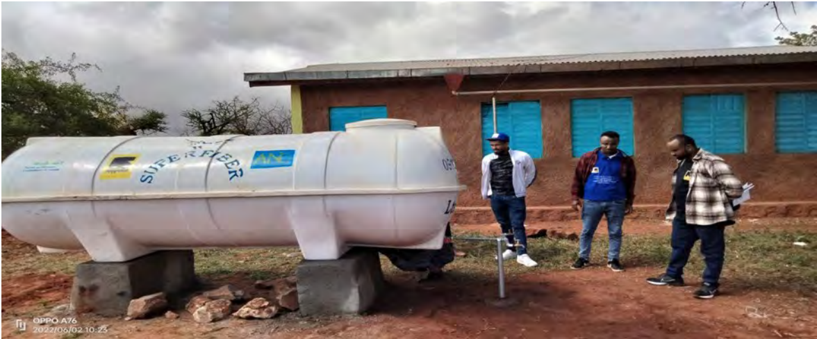
Fig. Install temporary water reservoirs
