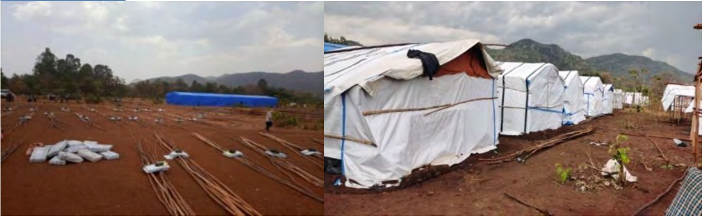
Fig: Constructed Emergency Shelters
